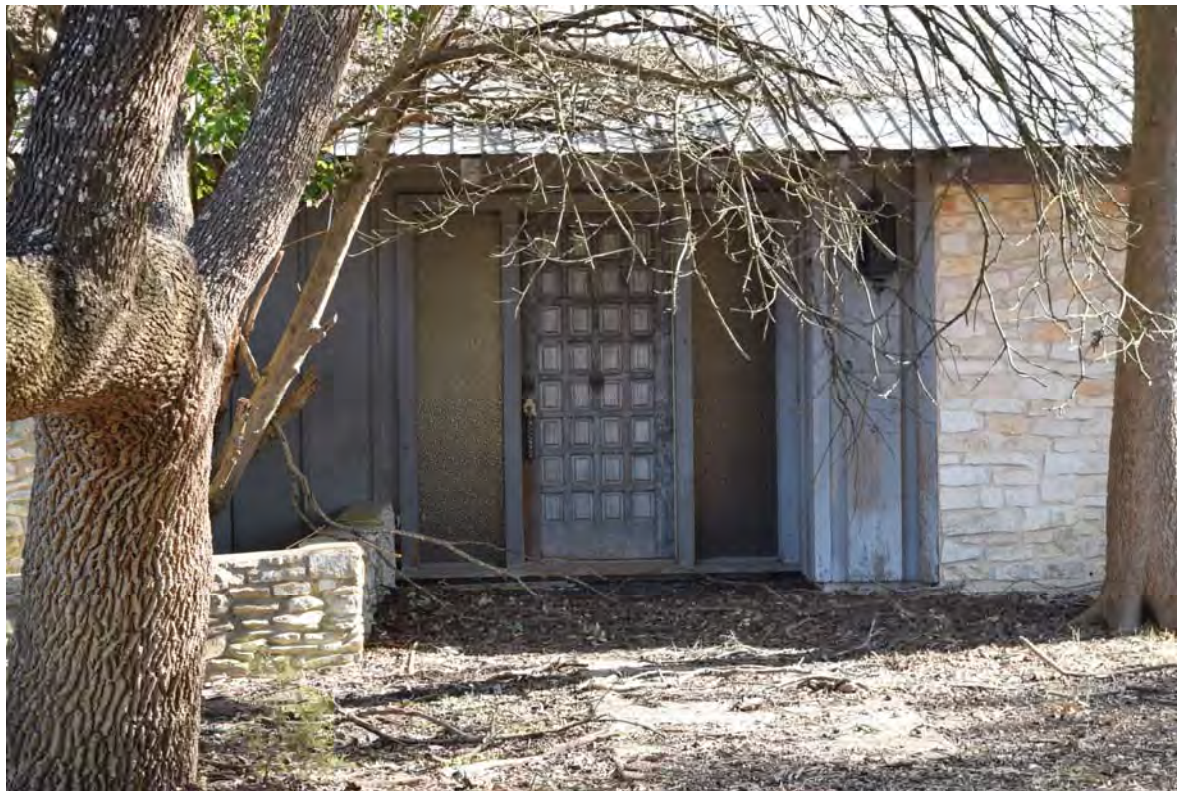
Close-up of primary entrance.
