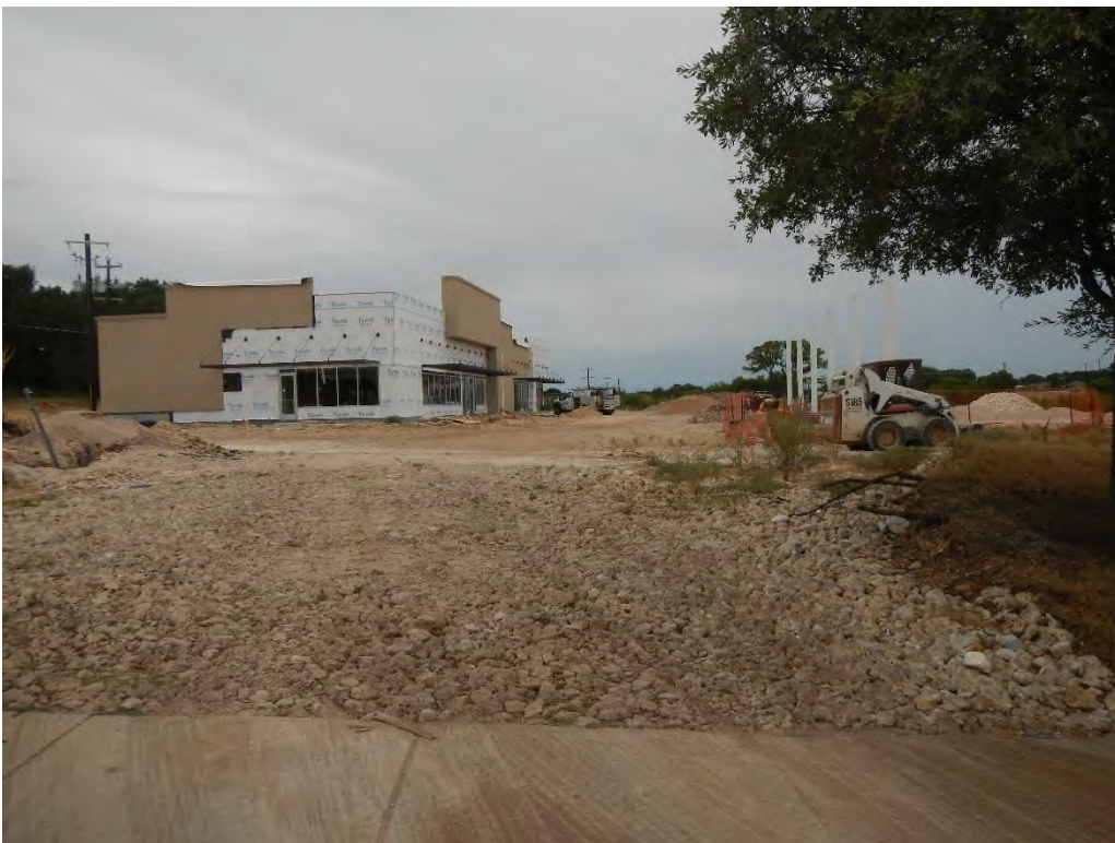
Photo 4: Figure 3 Site 4, future Chevron gas station, facing north.
