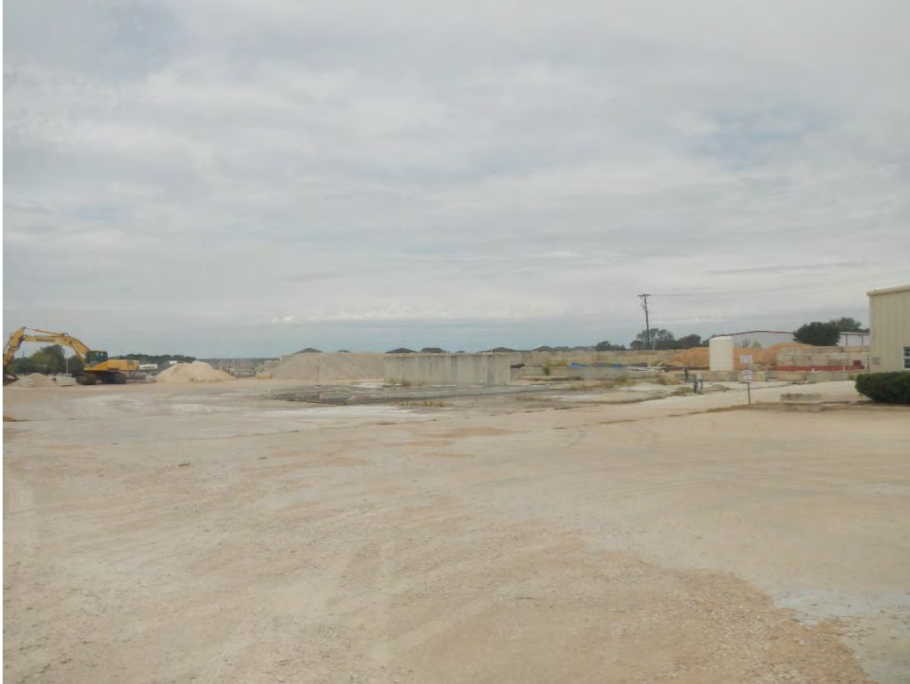
Photo 1: Figure 3 Site 1, Liberty Hill Plant, facing north.
