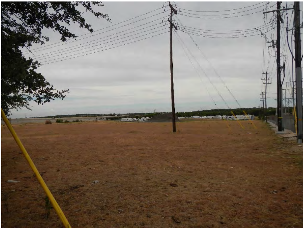
Photo 12: Stock pile located east of electrical substation, facing south.
