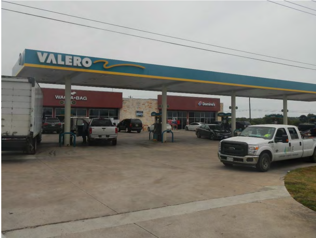
Photo 7: Figure 3 Site 7, Wag-A-Bag (active gas station), facing north.
