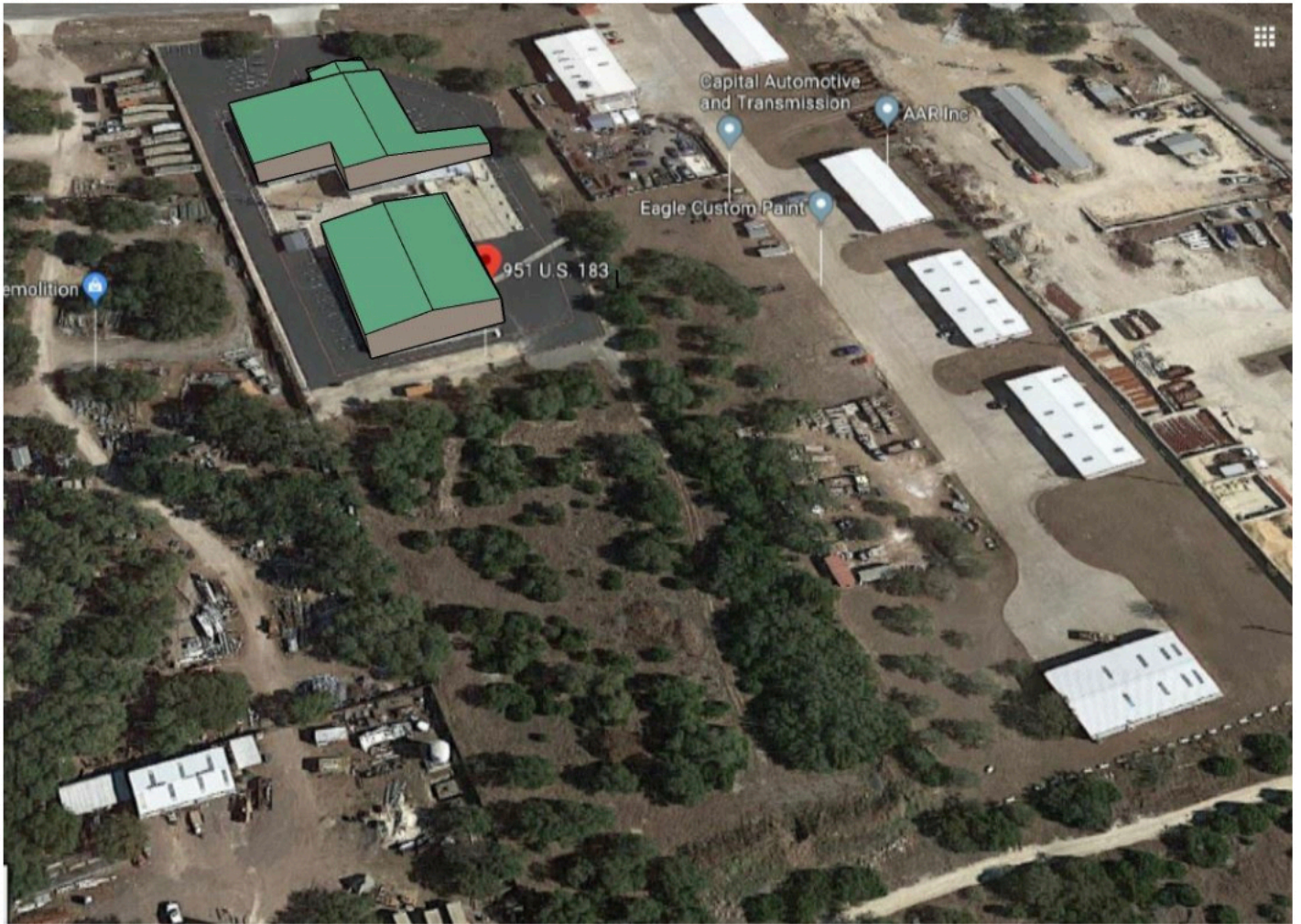
Facing East – Existing Conditions
