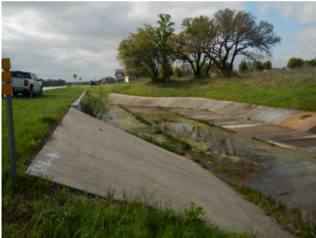
Photo 24: Stream crossing 2, west side of roadway, facing south, March 2017
