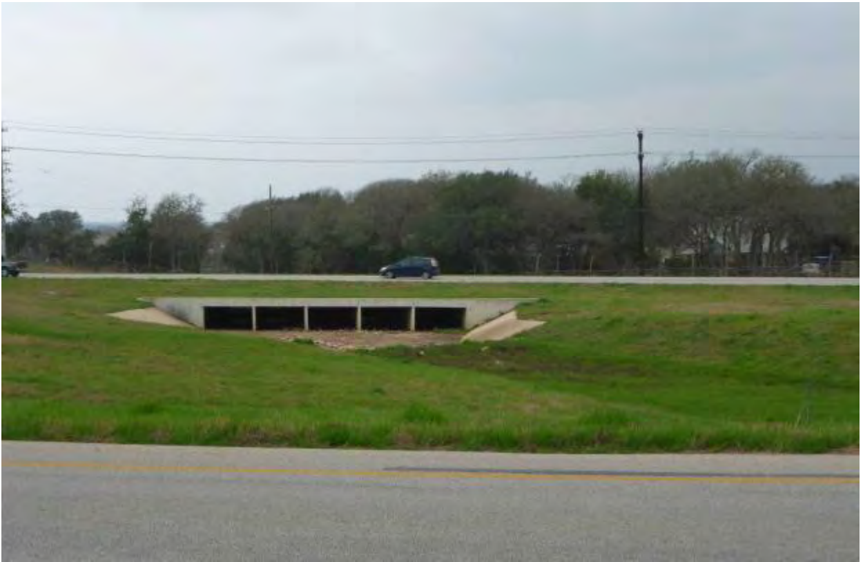
Photo 4: Culvert near Mourning Dove Lane, view facing southwest, February 2017
