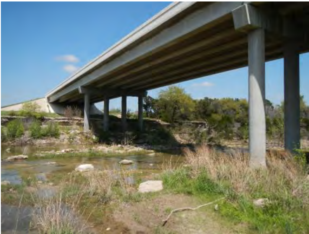
Photo 32: South Fork of the San Gabriel River, facing north, March 2017
