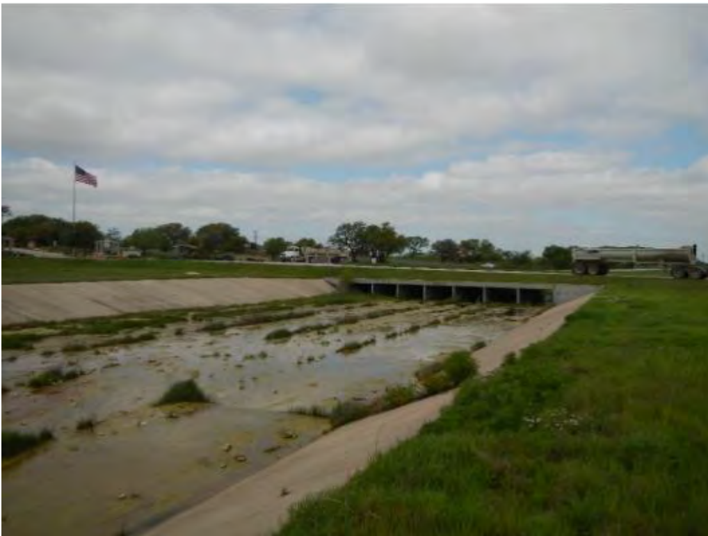
Photo 26: Stream crossing 2, median of US 183, facing northwest, March 2017
