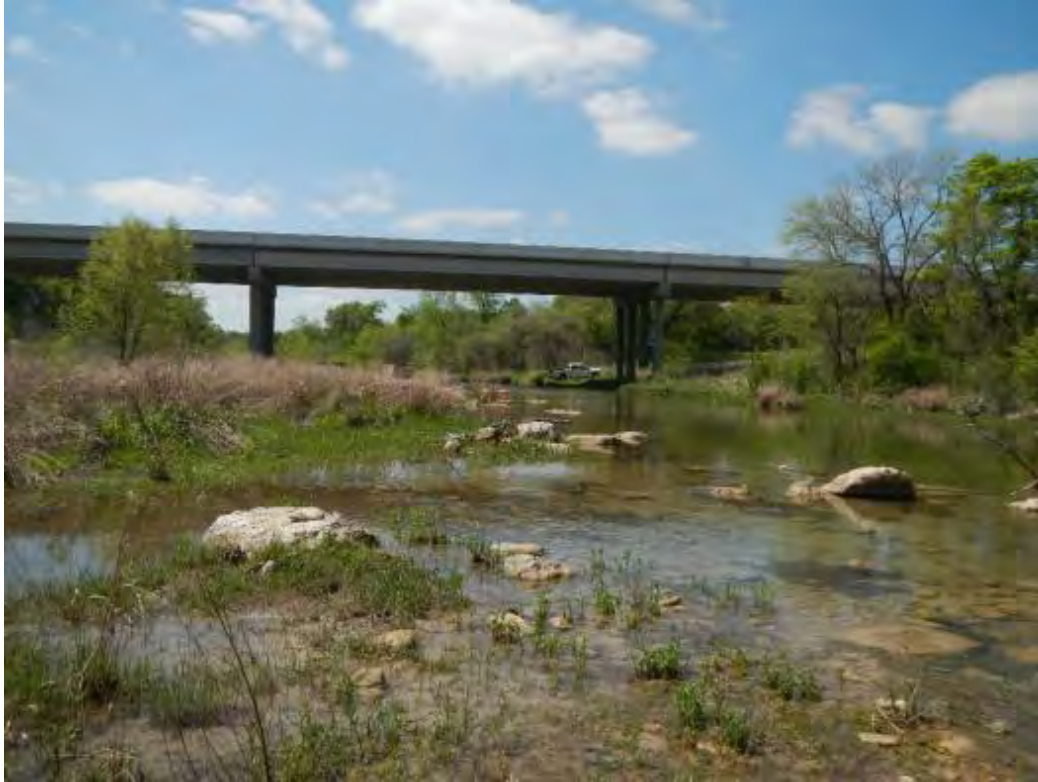
Photo 33: South Fork of the San Gabriel River, facing west, March 2017
