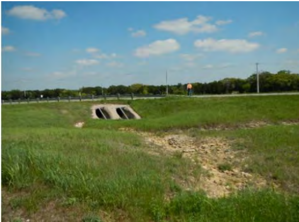
Photo 34: Stream crossing 4, west side of roadway, facing east, March 2017
