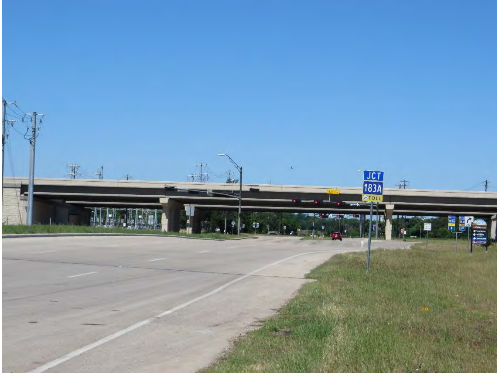
Photo 7: Existing grade separation at Hero Way and 183A, facing west southwest, May 2017
