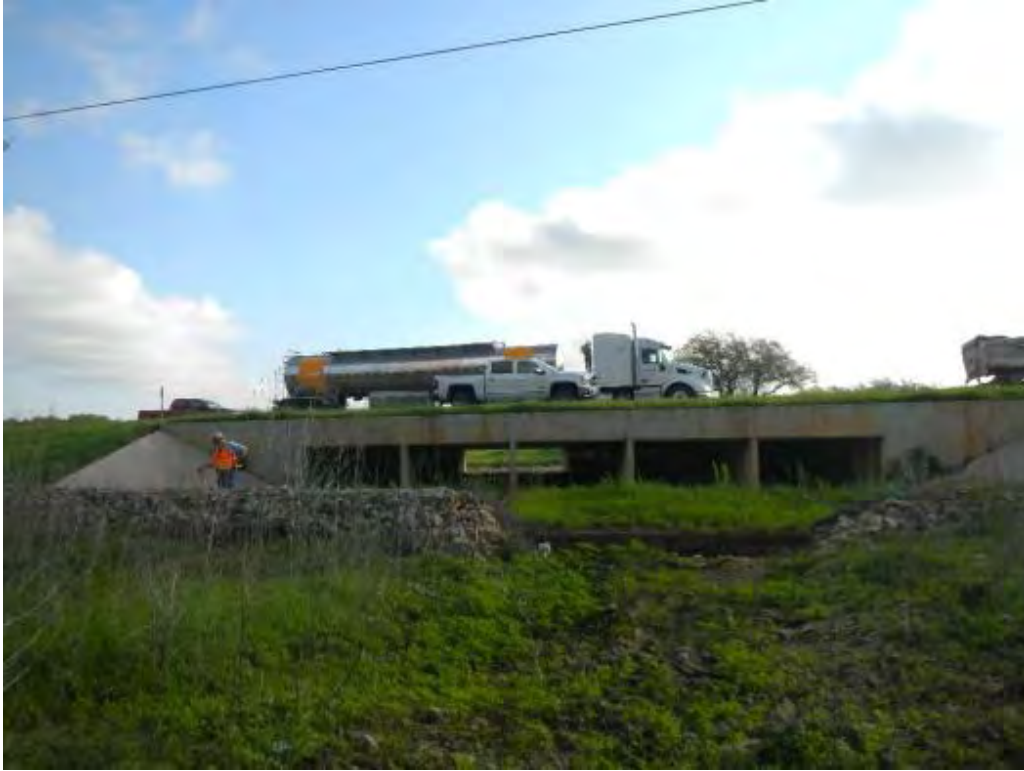
Photo 23: Stream crossing 1, facing southeast, March 2017
