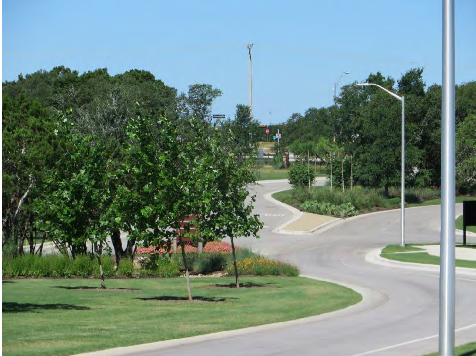
Photo 11: Bryson Ridge Trail/US 183 and 183A intersection (obscured by trees), viewed from Bryson Ridge Trail (approximately 880 feet east) in Bryson neighborhood, facing west, May 2017
