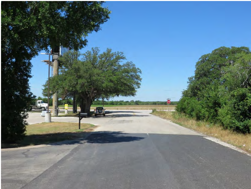
Photo 18: Planned Seward Junction Loop and US 183 intersection, facing west southwest, May 2017
