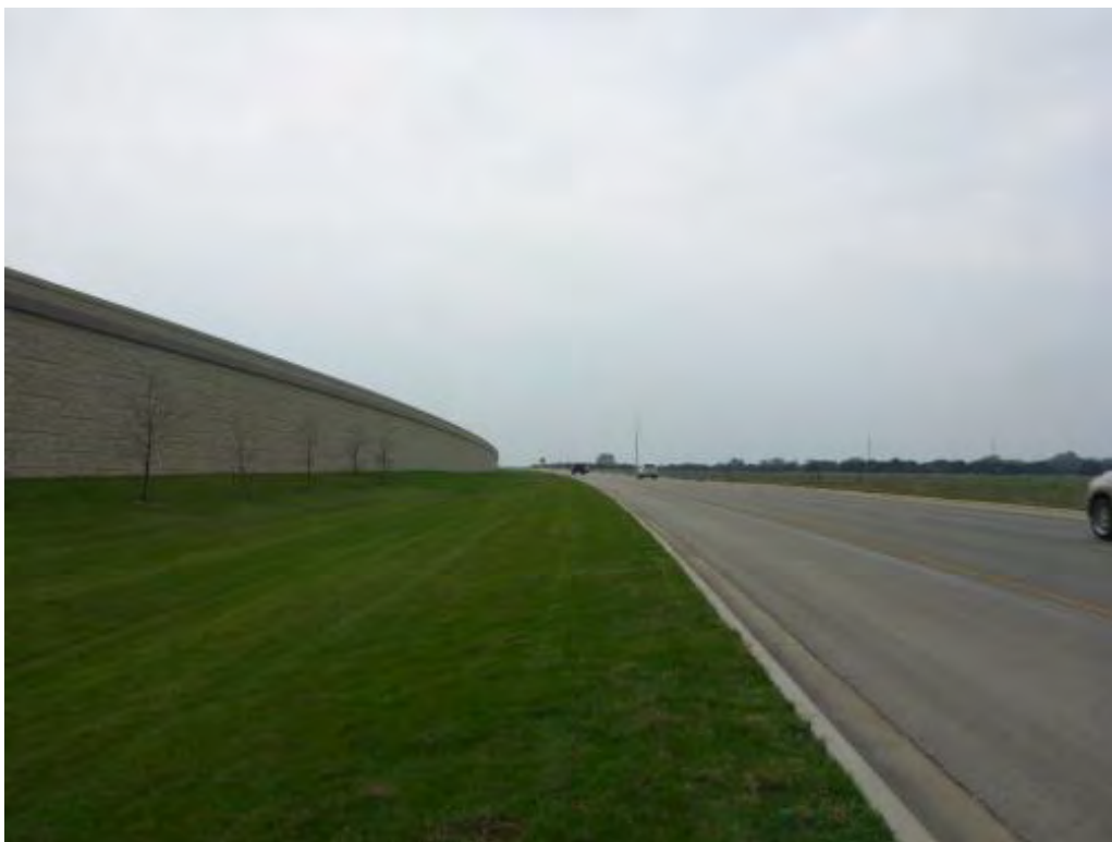
Photo 2: Southern project terminus, facing northwest, February 2017
